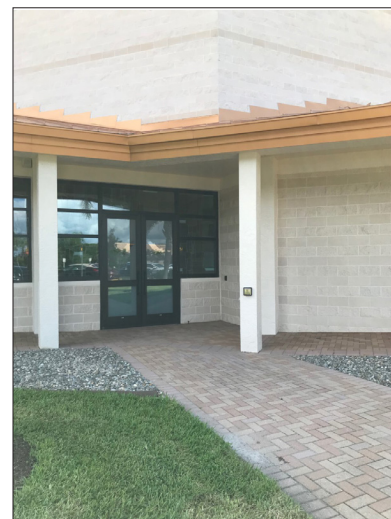
New Handicap Door Openers at Middle Lot Entrance
