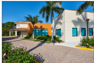
Exterior - Front Walkway
