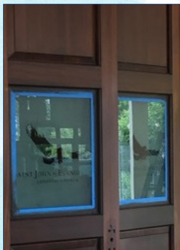
Front Doors are Original, but Have Been Stained to Match the Wood of the Church
