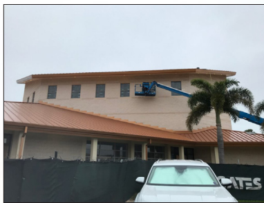
Exterior painting includes window frames
