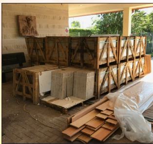
Flooring to be laid
