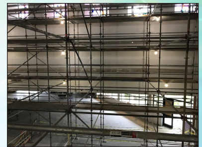
Scaffolding to put up multiple bands of marble
