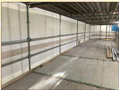
Marble arrives and flooring begins
