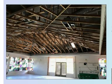
In removing the ceilings, it allows for us to repair structural and electrical issues that have caused problems in the back wings since the previous renovations. (left picture)
