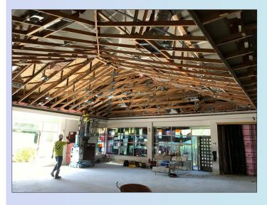
Water Intrusion through the vents damaged the drywall ceilings in the back wings. (left picture)
